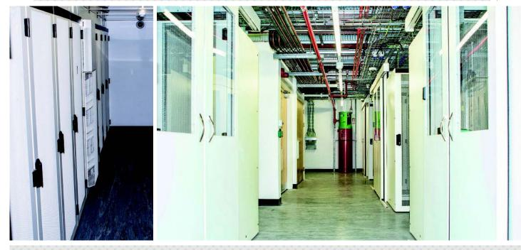
We have purpose built energy efficient aisle containment pods specifically for our co-location customers. Knurr row-based containment solutions can accommodate both standard and non-uniform hot & cold aisle configurations as required by your specification. Hot & cold aisle configuration separates the different air streams to improve data centre infrastructure efficiency. Physical barrier containment optimises this configuration for better cooling operation and higher efficiency.
